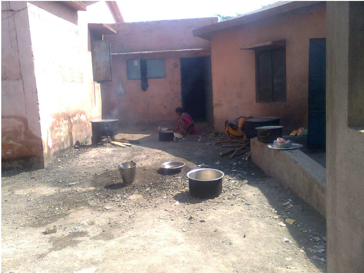
Kitchen shed: constructed but not in use
